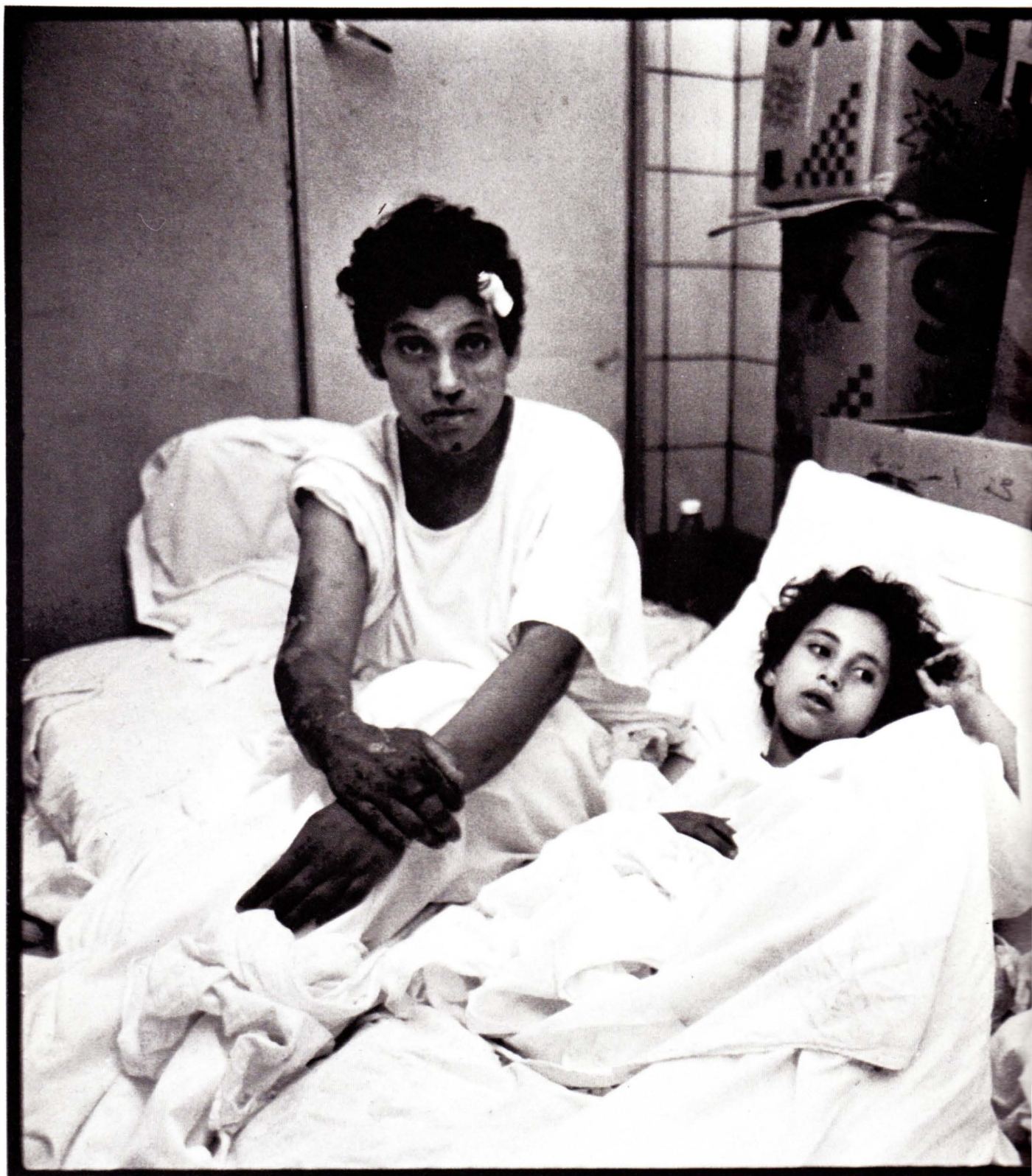
Basement of Barbir Hospital
